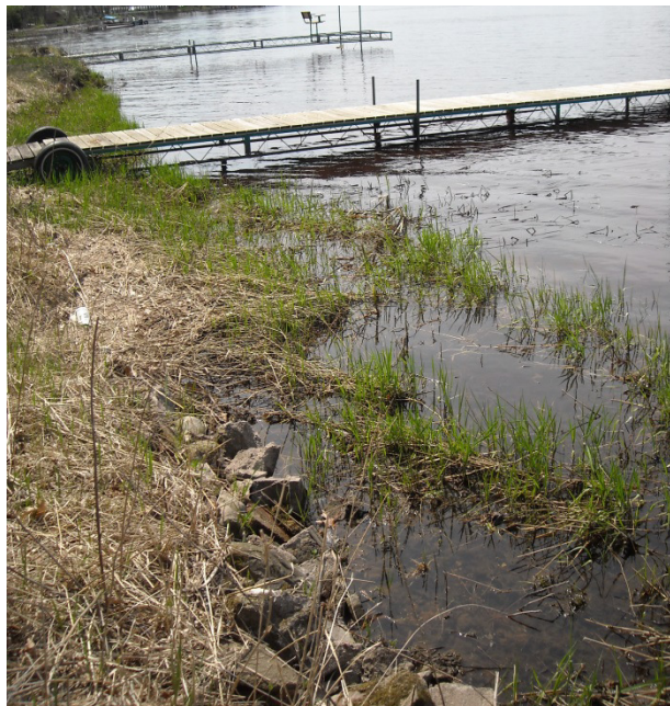
Erosion and invasive Reed Canary Grass
